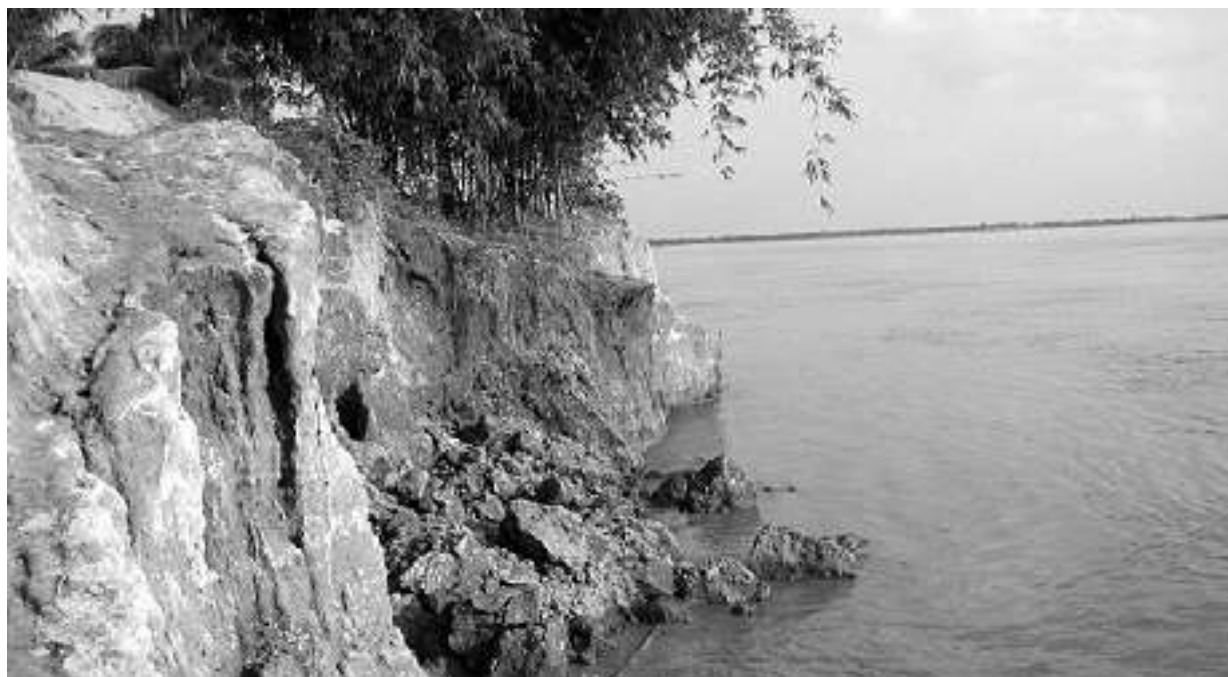
River erosion, a common phenomenon of Jamalpur area
